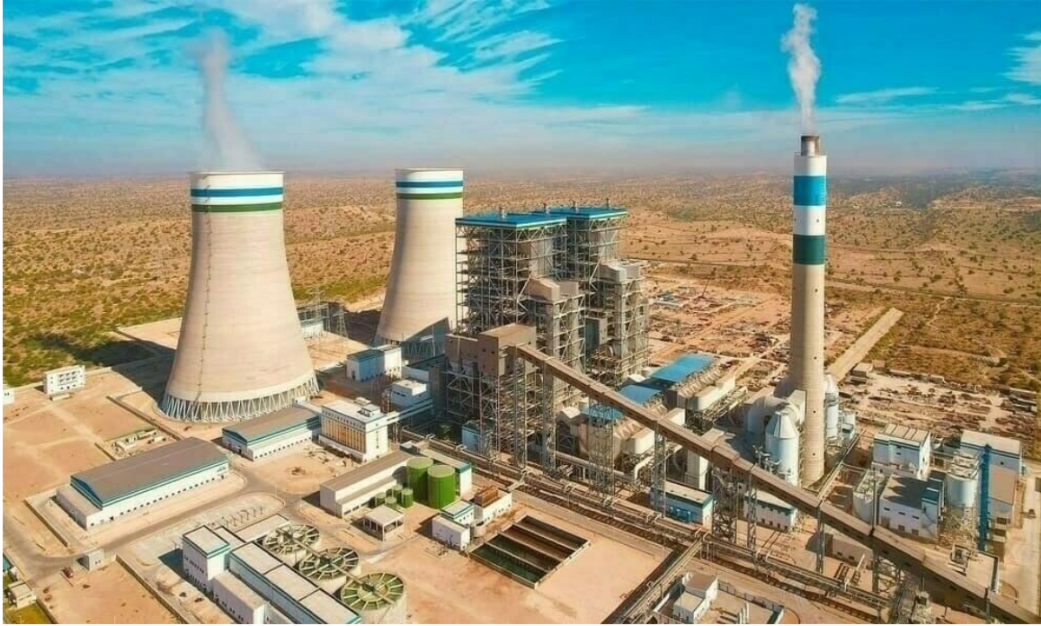
Figure 6 Jamshoro Coal-Fired Power Plant
