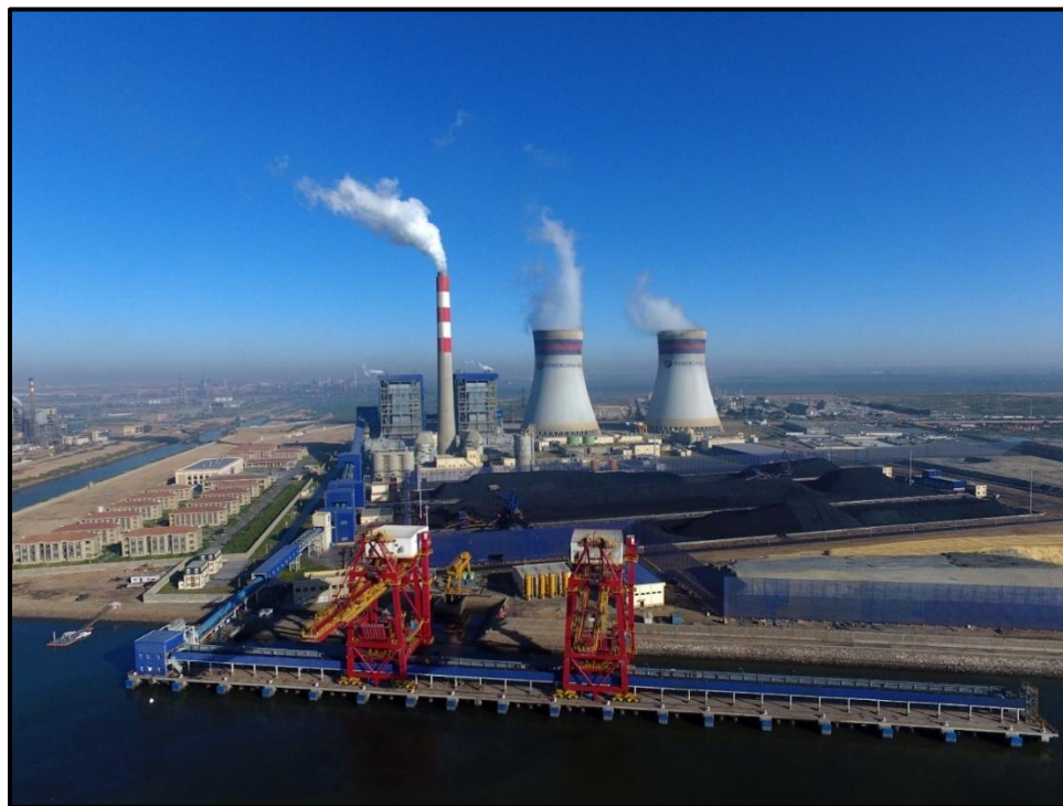
Figure 4 Coal-fired Power Plant at Port Qasim Karachi (Source: cpec.gov.pk/project )
