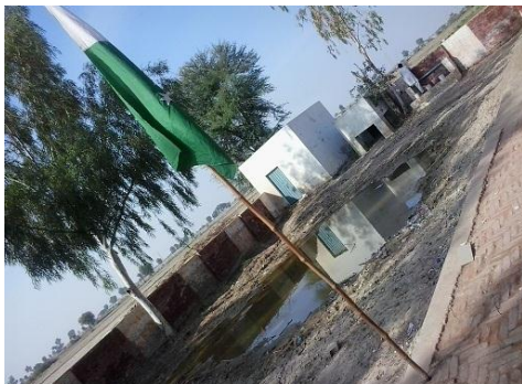
GBPS, BglaHidaya, Rojhan. Puddle of water stands in school
