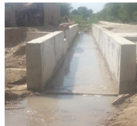
Figure 31: Concrete Water Course of Kousar Minor
